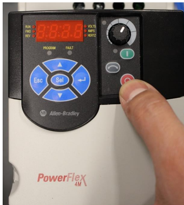
VFD Fault Reset Button
