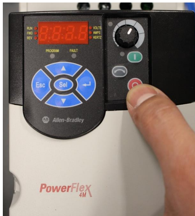
VFD Fault Reset Button
