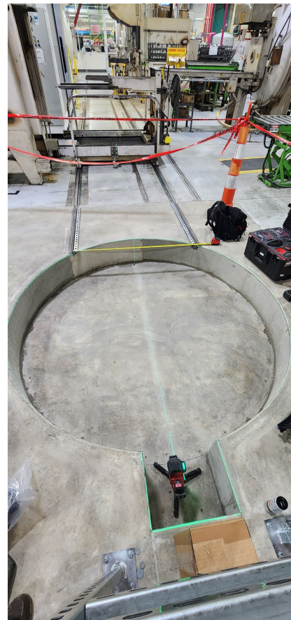
Laser alignment of the concrete pit against the existing floor tracks at the Cummins facility.
