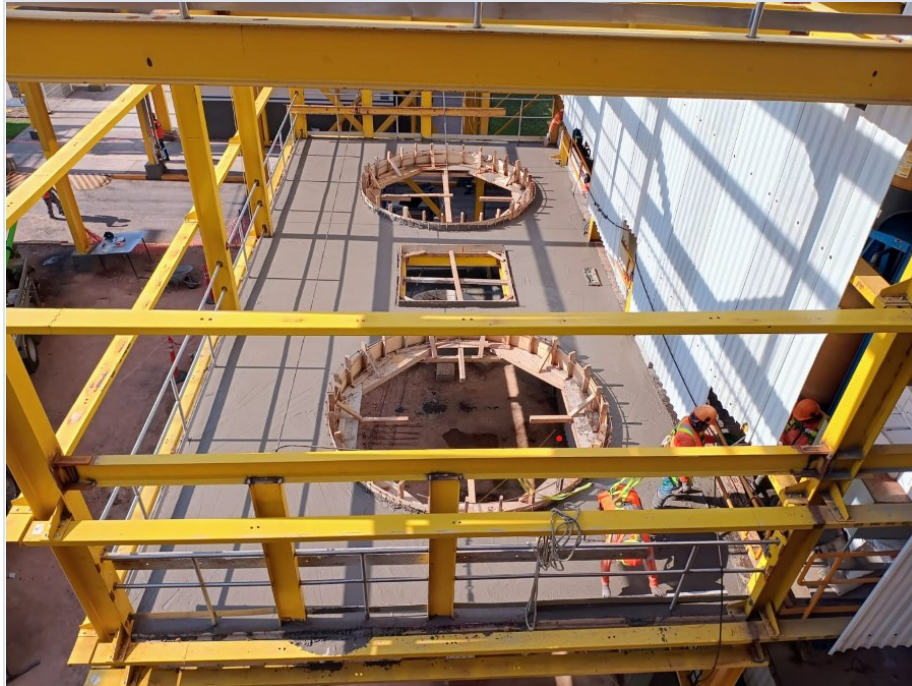
Foundation and pedestal preparation at the Querétaro facility ahead of erection.
